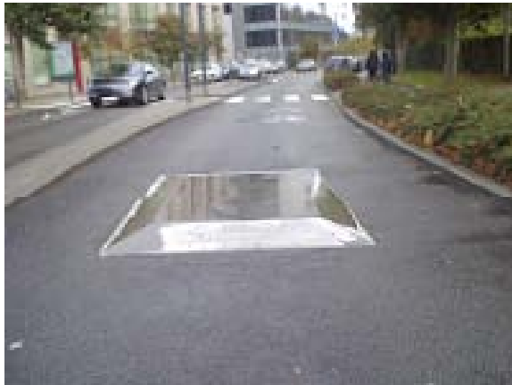
Fig. 6 Speed hump in urban areas. Source: Presto factsheet on traffic calming. Image source D. Dufour. 32
