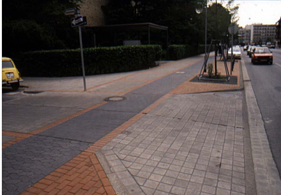
Fig. 26 Intersection between a bicycle path adjacent to a priority road and a minor road in Germany. Source: Planungsgemeinschaft Verkehr (PGV) and German Road Safety Council (DVR).
