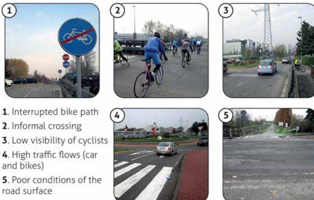
picture 06 Main cycling and safety constraints in the Alzaia Naviglio Pavese junction.
